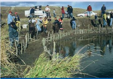
Wattle fence construction on West Nose Creek. The tools and techniques of bioengineering are quite simple, but the process can be labour intensive.
