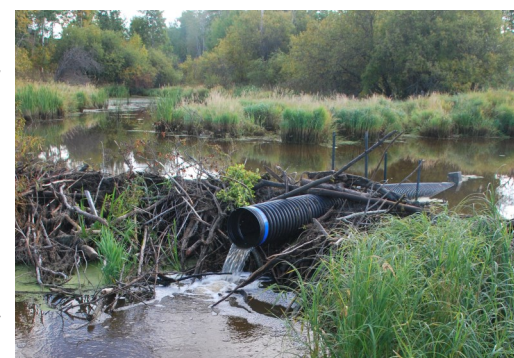
Photographs: Beaver pond leveller installation in Lac St Anne County.
