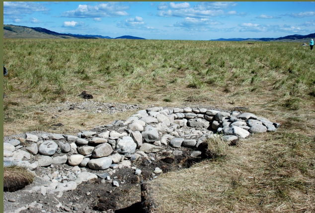
Photos: clockwise: Before photo of an actively eroding headcut; After photos of a Zuni bowl; log step down.
