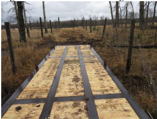
Windsor Creek Livestock Crossing Left: In Progress (Fall 2017) rig mat floor installed. Right: After installation (Winter 2018) complete with side panels. Photos: Adam Norris, MPWA.
