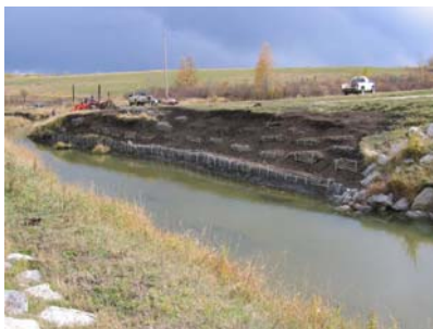
Site 2 (above) October 2007 – post bioengineering treatment including wattle fences, modified brush layers and live staking
