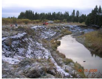
October 2009 – post bioengineering treatment including wattle fences & modified brush layers
