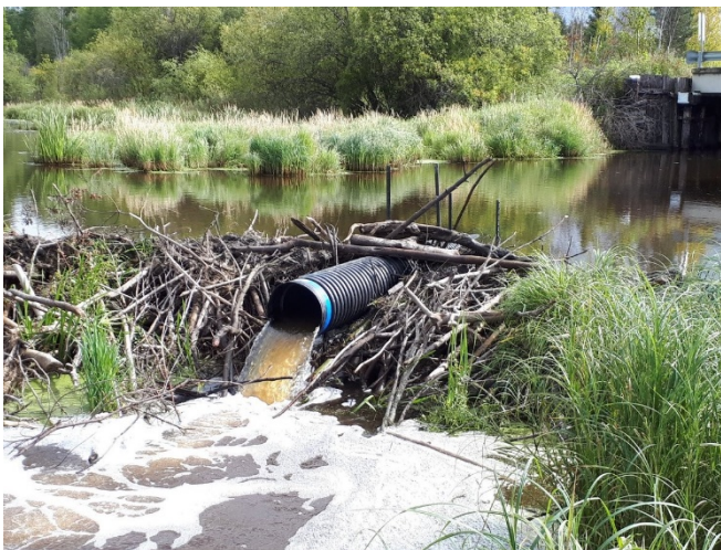
Pond levelling devices are installed in beaver dams, and can help regulate water level behind the dam
