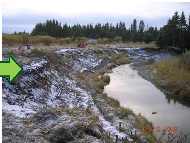
October 2009. Bearberry Creek site. Bioengineering treatment included wattle fences, modified brush layers and live staking.
