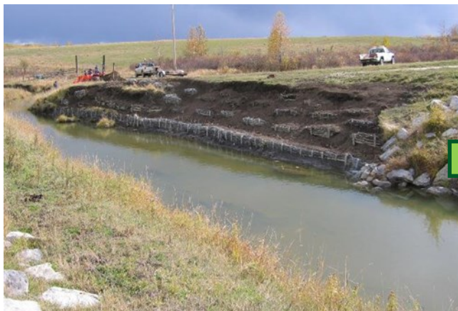
October 2007. Barry Creek site. Bioengineering treatment: wattle fence at water’s edge and modified brush layers along the bank slope.
