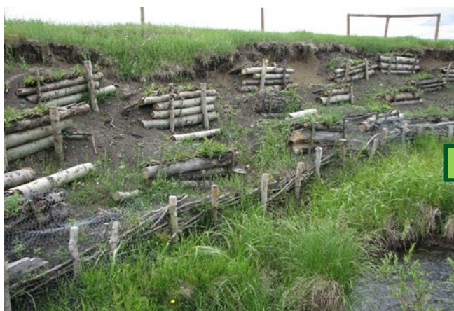
July 2009. Temple Creek site. One year post bioengineering treatment; wattle fences, modified brush layers and live staking. Rooting and shooting of willows from bioengineering structures is occurring.
