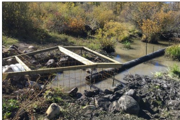
MD of Foothills culvert with modified exclusion fencing and pond leveller pipe. Site challenges: digging and removing large rocks near culvert which resulted in a very narrow exclusion cage to fit the site.
