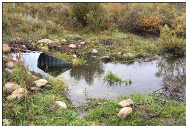
MD of Foothills culvert under road, before installation.
