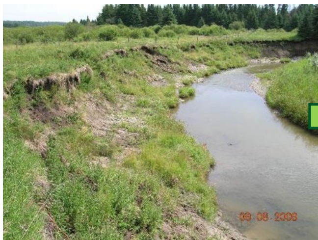
August 2006. Bearberry Creek site. Prior to bioengineering treatment. Slumping and eroding bank.
