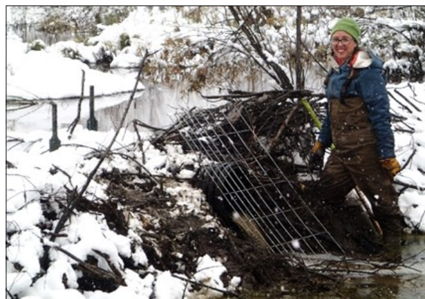
After a messy job of clearing out mud and sticks from the pipe, we installed an angled panel "cage" over the outlet of the pipe – after thoroughly covering the sides and front with sticks to prevent the beavers from further accessing the pipe.
