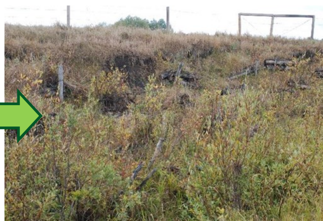
September 2017. Temple Creek site. Willow has regenerated and revegetated the site. Slumping and erosion have ceased.
