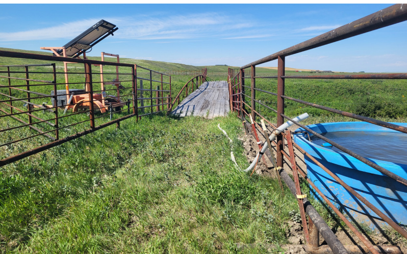
A new bridge to cross the stream is in place at Crowfoot Creek. In addition, a solar powered livestock watering system provides water away from the streambanks, as part of their larger management project started in 2021.
