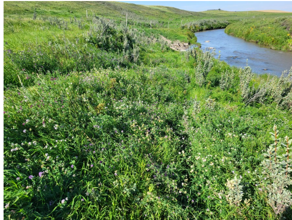
CRO39_2025. Since the 2021 photo was captured (image to the left), the livestock trail has revegetated. In addition to earlier management changes at this site, including livestock exclusion fencing and alternative watering options, a new elevated bridge crossing is in place to allow access for livestock to pastures on both sides of the creek and prevent stream channel and bank impacts. (Photo: RHIP39CRO017)
