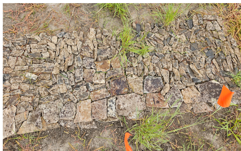
Steps to implement when building a one rock dam. 1) Remove objects in the way and flatten. 2) Carefully select rocks for footer. 3) Ensure footer is flat and embedded. 4) Add rows until level.
