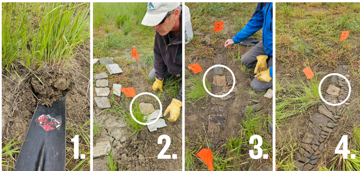
Steps to implement when building a one rock dam. 1) Remove objects in the way and flatten. 2) Carefully select rocks for footer. 3) Ensure footer is flat and embedded. 4) Add rows until level.
