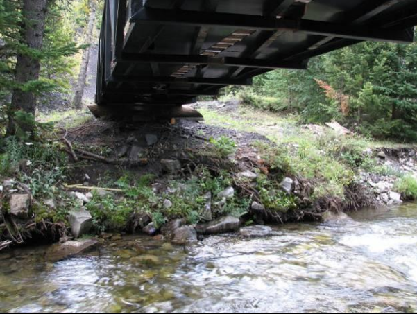
LEFT BANK, AT NEW QUAD BRIDGE CROSSING (Photographer: J. Melsted, Catalogue No: RHIP03GOL005)
