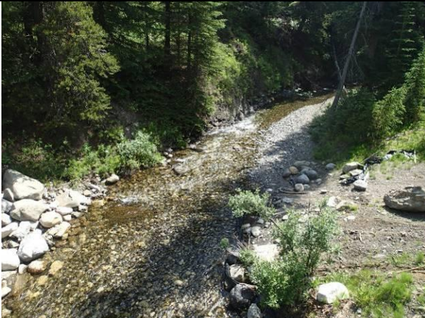
STREAM CROSSING LEFT AND RIGHT BANK, VIEW DOWNSTREAM FROM BRIDGE
