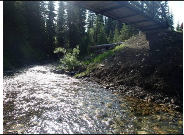
STREAM CROSSING RIGHT BANK
