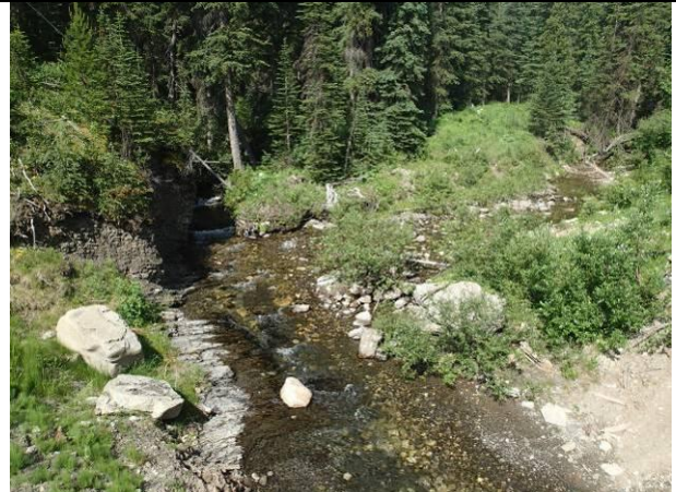
STREAM CROSSING LEFT AND RIGHT BANK, VIEW UPSTREAM FROM BRIDGE.
