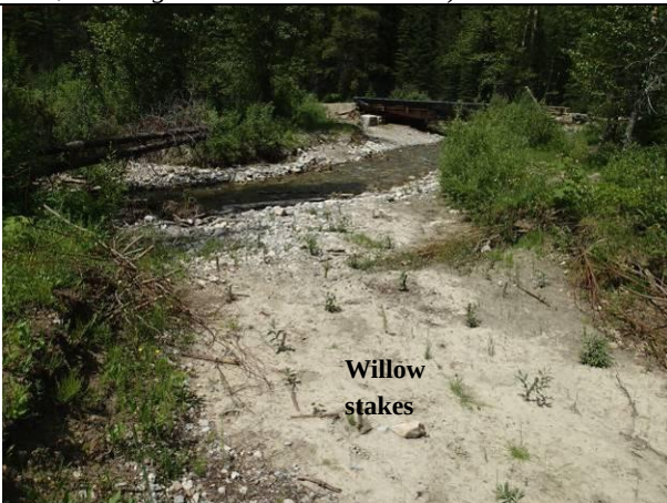
WILLOW PLANTINGS IN FOREGROUND, VIEW UPSTREAM TO TEMPORARY LOGGING BRIDGE (Photographer: A. Sarrazin, Catalogue No: RHIP03ALL002)
