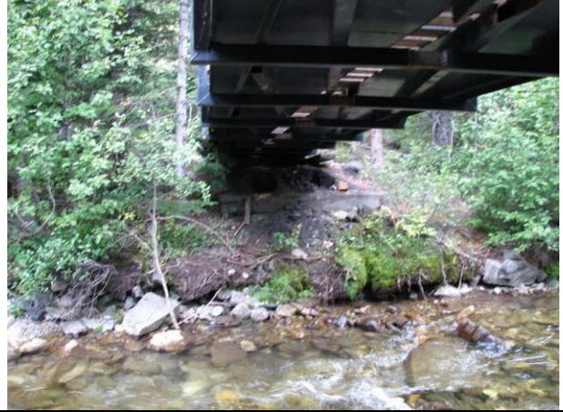
RIGHT BANK, AT NEW QUAD BRIDGE CROSSING (Photographer: J. Melsted, Catalogue No: RHIP03GOL006)
