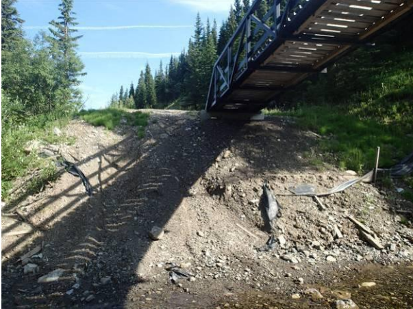
STREAM CROSSING LEFT BANK.
