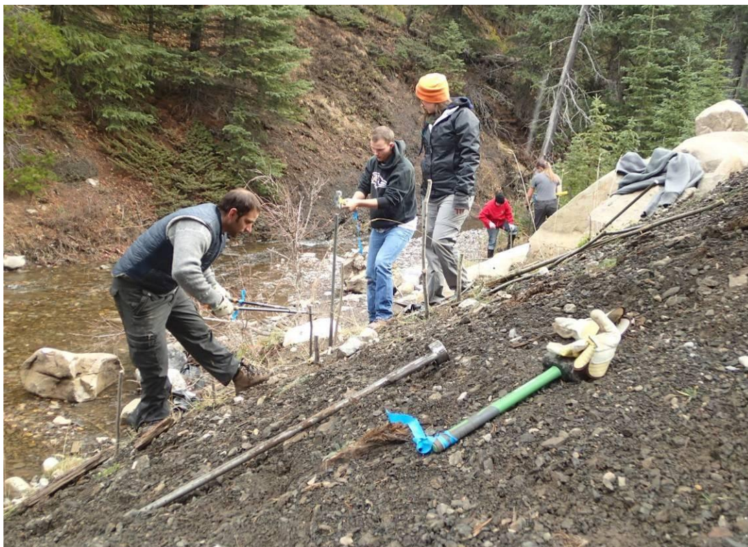
Smith Creek (SMT2) riparian planting project, October 24, 2014. Live willow and balsam poplar stakes were installed on the steep approach slopes adjacent to the quad bridge to help stabilize and reduce bank erosion.
