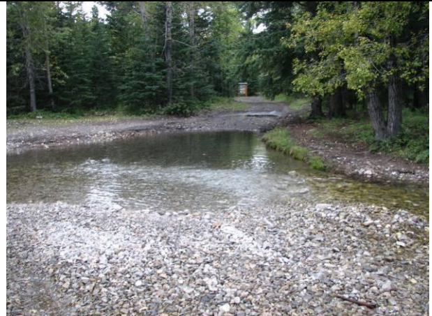
A forded truck trail crossing upstream of the new quad bridge. (Photographer: M. Plemel, Catalogue No: RHIP01GRE005)
