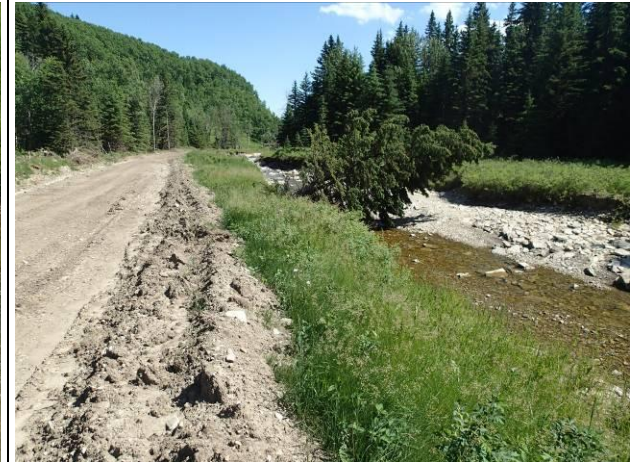
Photo n: A logging access road running parallel to Trout Creek has created a source of sediment and contributed to soil compaction and loss of vegetation cover. (Photographer: A. Sarrazin, Catalogue No: RHIP01TRO033)
