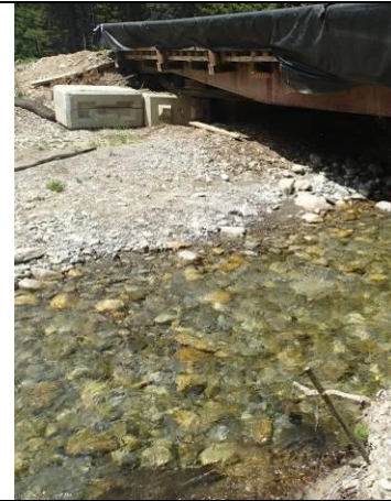
FORDED STREAM CROSSING RIGHT BANK DOWNSTREAM OF TEMPORARY LOGGING BRIDGE (Photographer: A. Sarrazin, Catalogue No: RHIP03ALL007)
