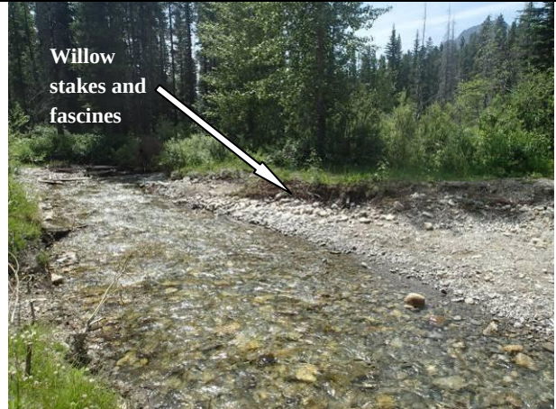
FORDED STREAM CROSSING VIEW TO RIGHT BANK DOWNSTREAM OF TEMPORARY LOGGING BRIDGE (Photographer: A. Sarrazin, Catalogue No: RHIP03ALL010)
