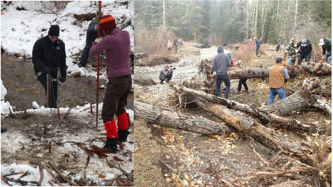
Allison Creek (ALL3) riparian planting project – November 8, 2013 (Left) and October 24, 2014 (Right). Balsam poplar, willow and red-osier dogwood live stakes were installed in both years. In 2013 and 2014, large woody debris was placed on the left bank by Spray Lake Sawmills to prevent OHVs from fording through the creek.
