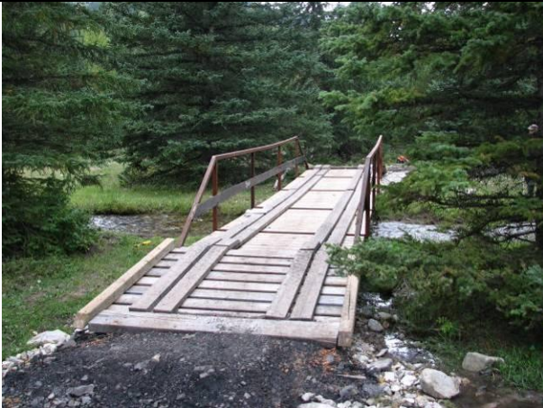
NEW QUAD BRIDGE APPROACH (VIEW FROM LEFT BANK TO RIGHT BANK) (Photographer: M. Plemel, Catalogue No: RHIP01GRE006)
