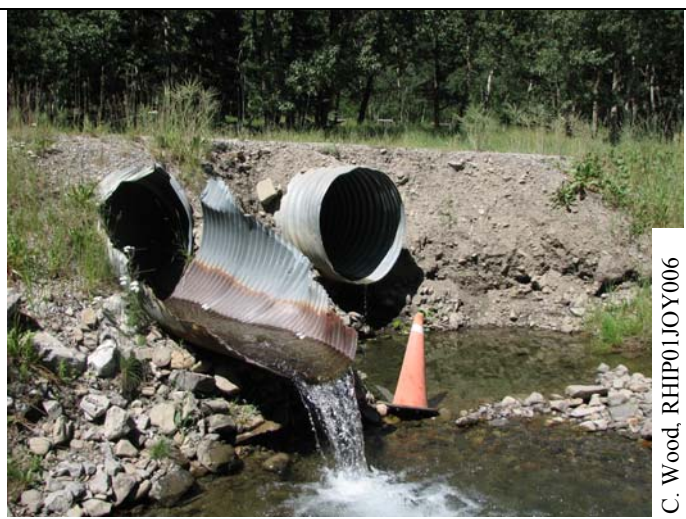
Photo x: Hanging culvert (barrier to fish passage) at the downstream end of JOY1.
